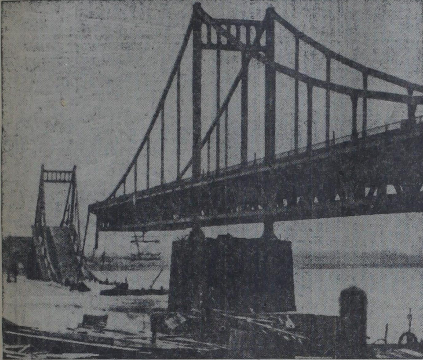
HITLER BRIDGE —Only twisted wreckage remains of the Adolf Hitler bridge, which crosses the Rhine river at Uerdingen. The middle span of the bridge was blown up as retreating Nazis made their way to the east bank at this point. (Signal Corps photo).
