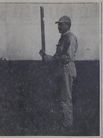
For those who may wonder what's going on, Brock is using a farm level to take a reading across the field of Walt Mabry near the Hub. Jim Terrell, right, holds a "target" for the level. As the target is moved up or down the slide, numbers indicate the rise or fall of the portion of the field on which he may be standing. The two men are sighting in an irrigation ditch line for Mabry.
