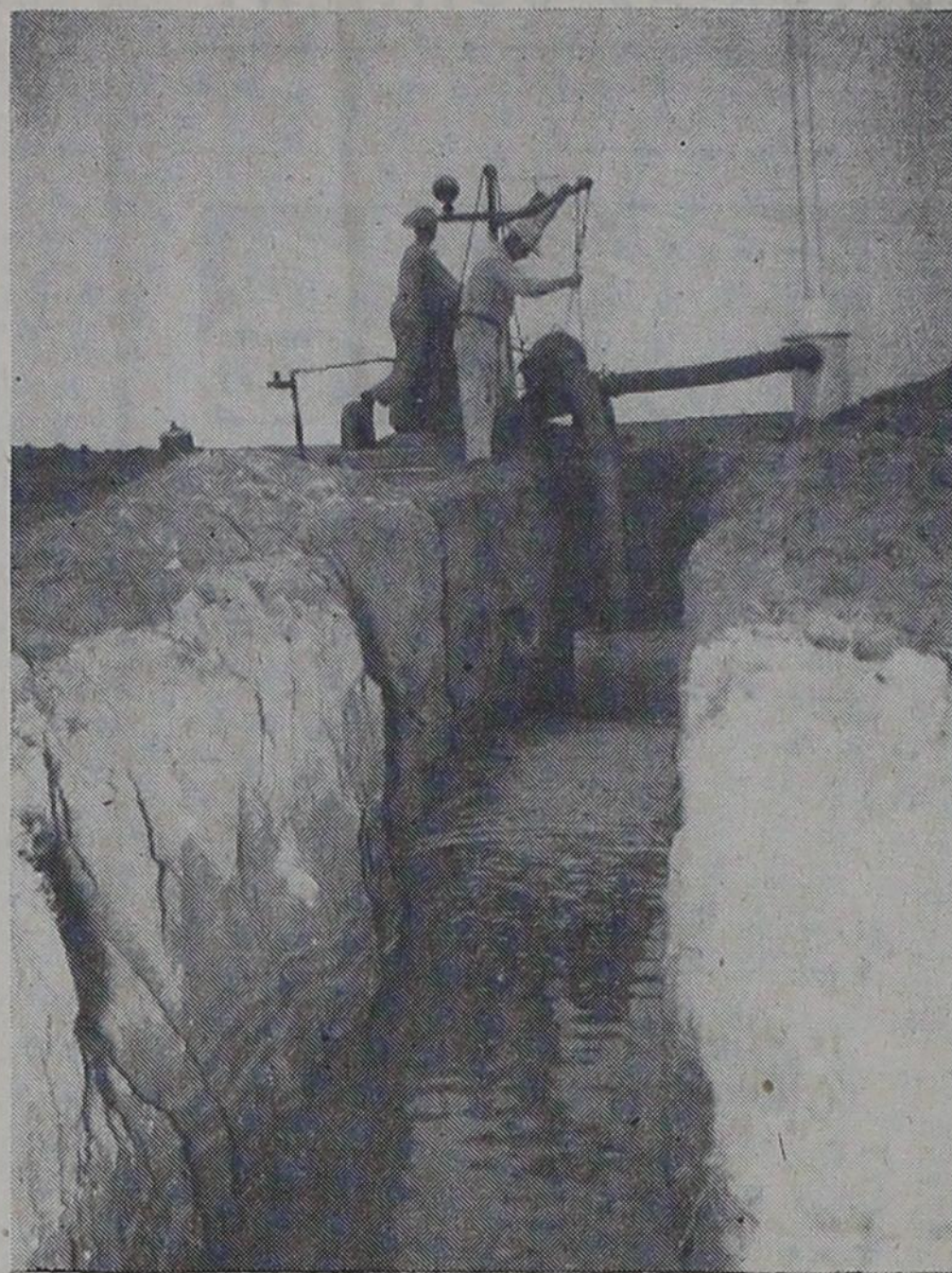
It is through this ditch that water from a surface lake on the Archie McCutchan place flows to a pumping station at the lower end of one of McCutchan's fields. It is then raised and forced uphill to irrigate bench levelled land.
