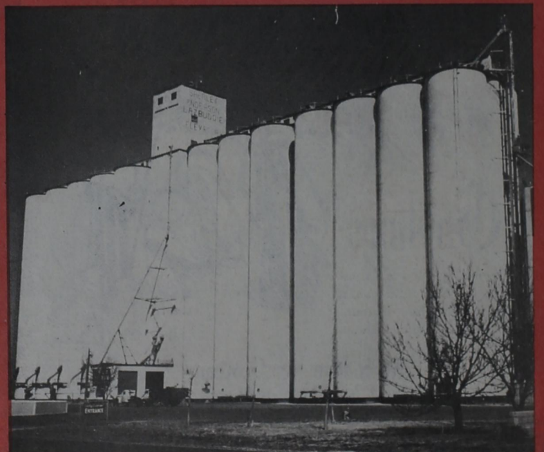
Sherley - Anderson Lazbuddie Elevator
