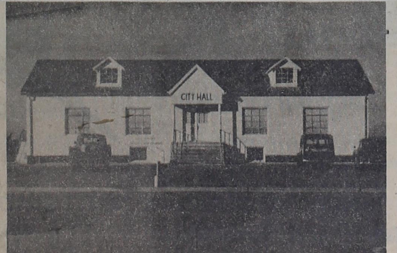
NEW PAINT--Farwell city hall is glistening with a new paint job, including red trimming. The work was done by Utzman and Fought of Farwell.
