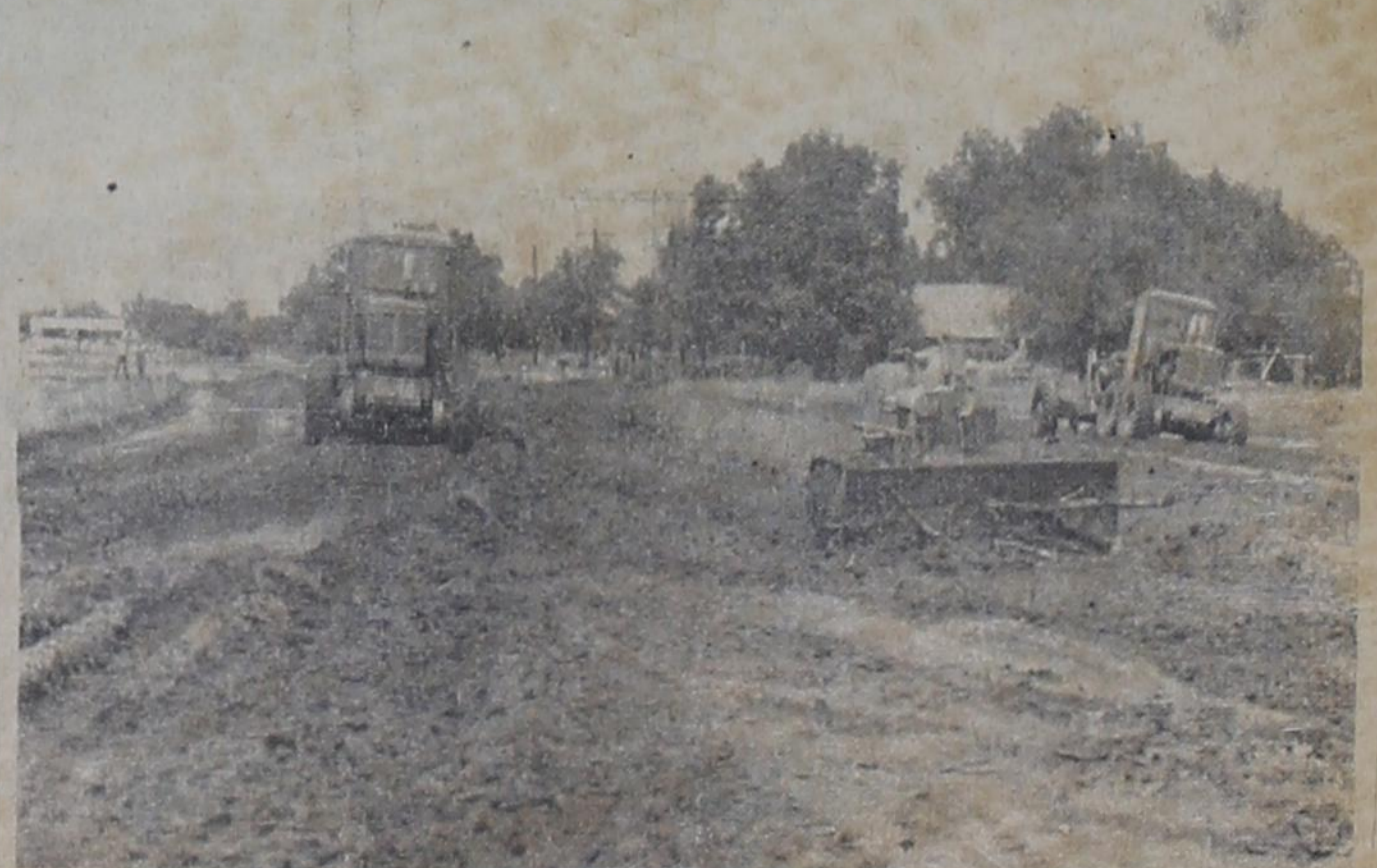
IN A SEA OF MUD, this sturdy bulldozer wallows through a boggy assignment for the Texas Highway Department on Ninth Street, Farwell. Construction started Monday and over an inch of rain fell that afternoon and night. Tuesday, however, work went right ahead. The "loop" is expected to take about a month to build. Below, two motor erasers join the bulldozer in dirt moving.
