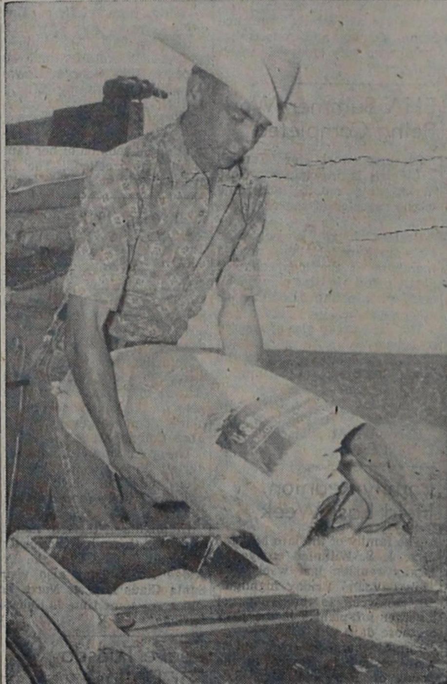
Leon Richards, Highway Department employee, empties a sack of soil sterilant into a waiting spreader. Borasuc is the chemical being used by the state to control bindweed.
