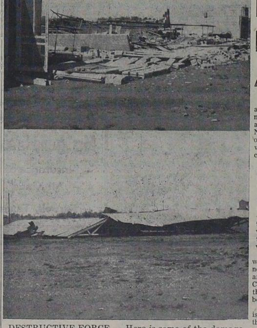
DESTRUCTIVE FORCE - Here is some of the damage who left the Gin office at 4 p.m., which was caused Monday by the strong wind. The top says it must have been done bepicture shows what was left of the west portion of a concrete-tile building at Nickels' Gin in Farwell and the bottom picture shows the roof which was blown off, landing about a 100 feet north of the structure. One wall of the building had been blown in by wind several weeks
