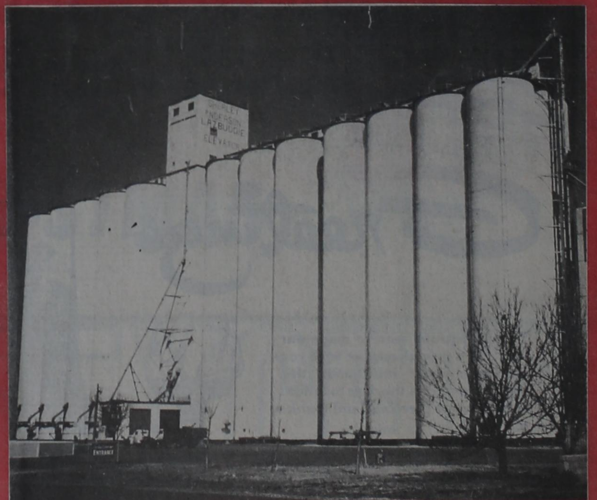
Sherley - Anderson Lazbuddie Elevator
