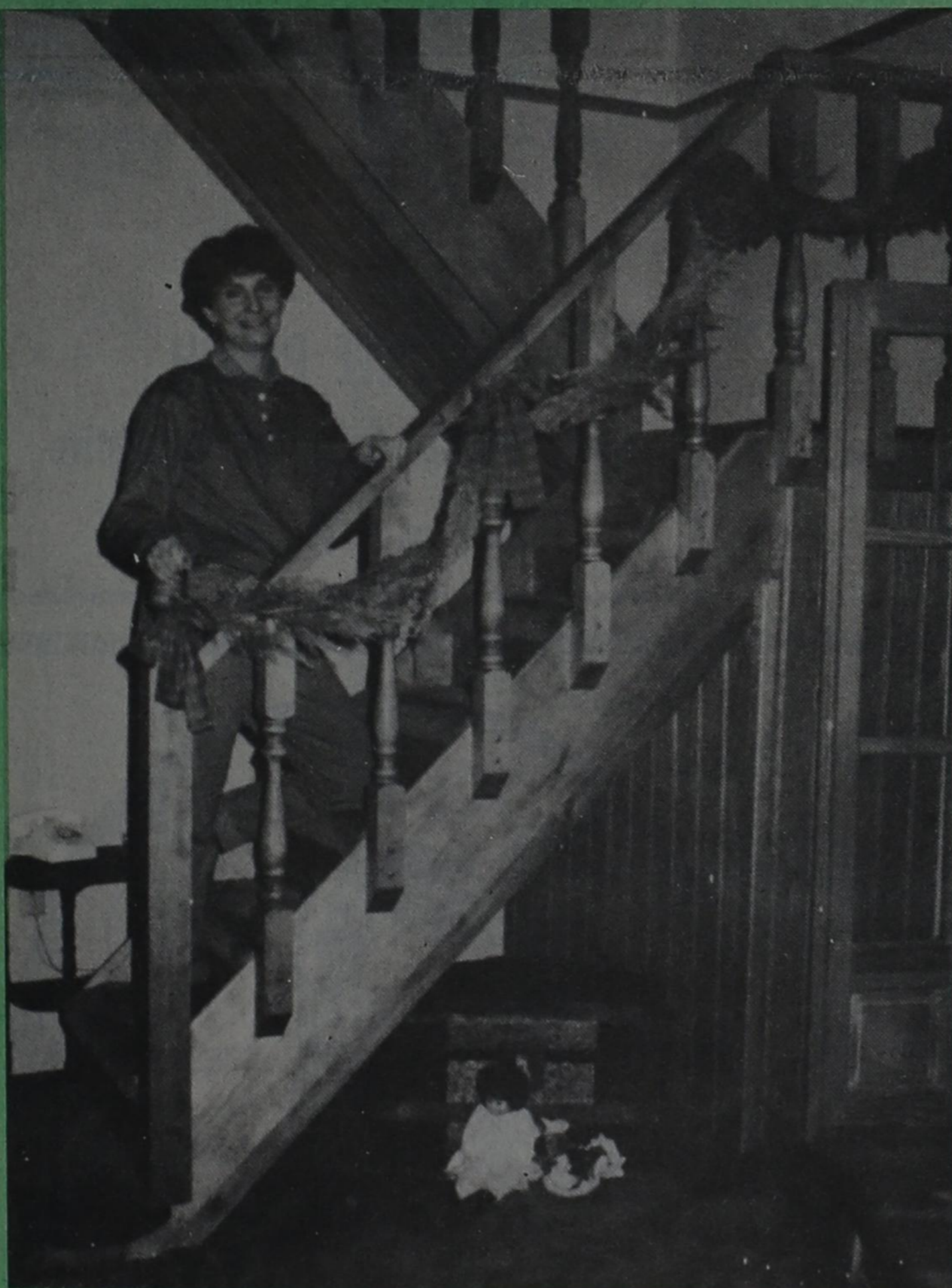
Joey stands on the staircase that they rebuilt which leads to the attic.
