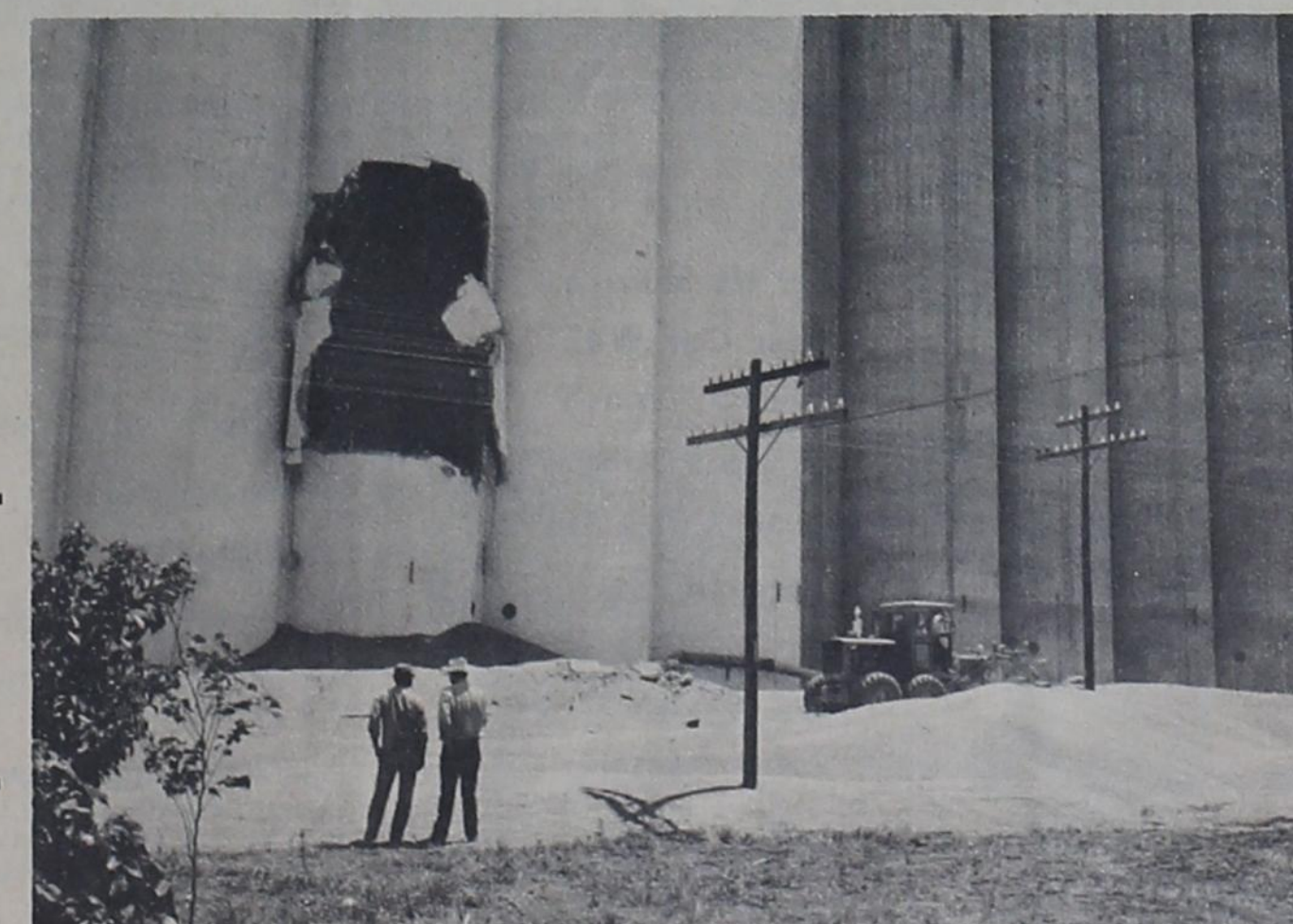
WHO KNOWS what happened Saturday morning when some 40,000 bushels of wheat came tumbling down from Sherley-Anderson Lariat Grain Co. through a hole approximately 30 feet long. Asa Smith, elevator manager, said "The first thing we knew a cloud of dust rose--no noise, and the grain came pouring out." Grain was being moved from one tank to another tank at time of the incident. Smith stated that the loss of grain would be much less than would be expected and repairs on the elevator would be completed in ample time for the fall grain harvest. The grain had been moved from the railroad tracks which ran adjacent to the elevator by 1 p.m. Saturday and extra help came to pick up the grain. Clean-up operations were being completed Monday morning.
