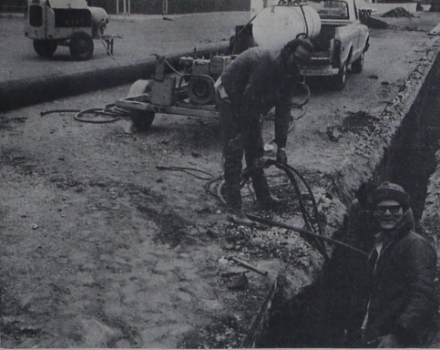
WATER WORKS NEAR COMPLETION - A major water works expansion program is nearing completion in Farwell. The work is being done by Sheets & Sheets Trenching and Welding Service of Texico. Pictured here are three workmen as they cut the last ditch under Highway 70-84 to make the final water connection. The drilling under the highway is being done with a hydrodrill, and the 16 inch water line in the background will be installed. Local water officials have commended the work as done by the local firm. Pictured are: facing camera, Roland Gotforth and in the ditch with him is Johnny Hammit. Also shown is another workman, George Venter.
