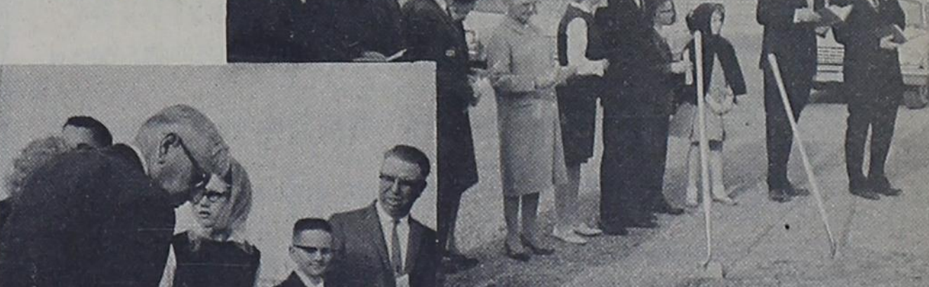
Groundbreaking for the new sanctuary of Hamlin Memorial Methodist Church was held Sunday. On the left, J. R. Thornton, turns a spade of dirt. Other participants in the service are pictured in the upper panel. Rev. W. C. Strickland, pastor, and Rev. B. C. Goodwin of Portales, presided.
