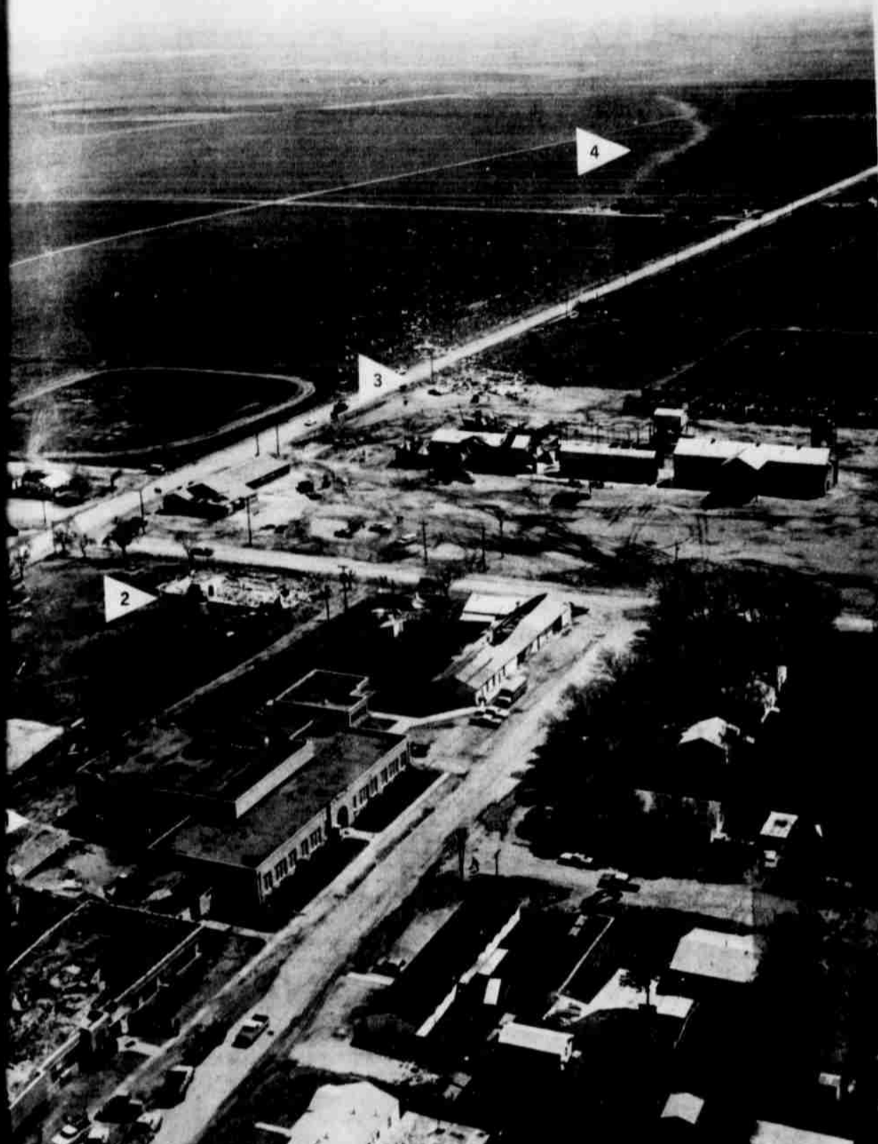
PATH OF THE tornado that hit Whitharral Friday evening is plainly visible in this aerial photo. In the upper left is the elementary school building which is damaged beyond repair. The structure just below number one is the cafeteria where portions of the roof in the cafeteria and stage were torn off. Arrow number one points toward the gymnasium. The topless shell is the girls' dressing rooms; the boys' dressing rooms are to the west side and the west and north ends of the gym are demolished. Number two arrow is the remains of the ag shop. The third arrow is the rubble left where the Joe Chavez family lived and arrow four shows the definite path cut by the tornado as it traveled northeast toward Anton. (Photo by Bill Turner, from the film flown by P&H Flying Service.)
