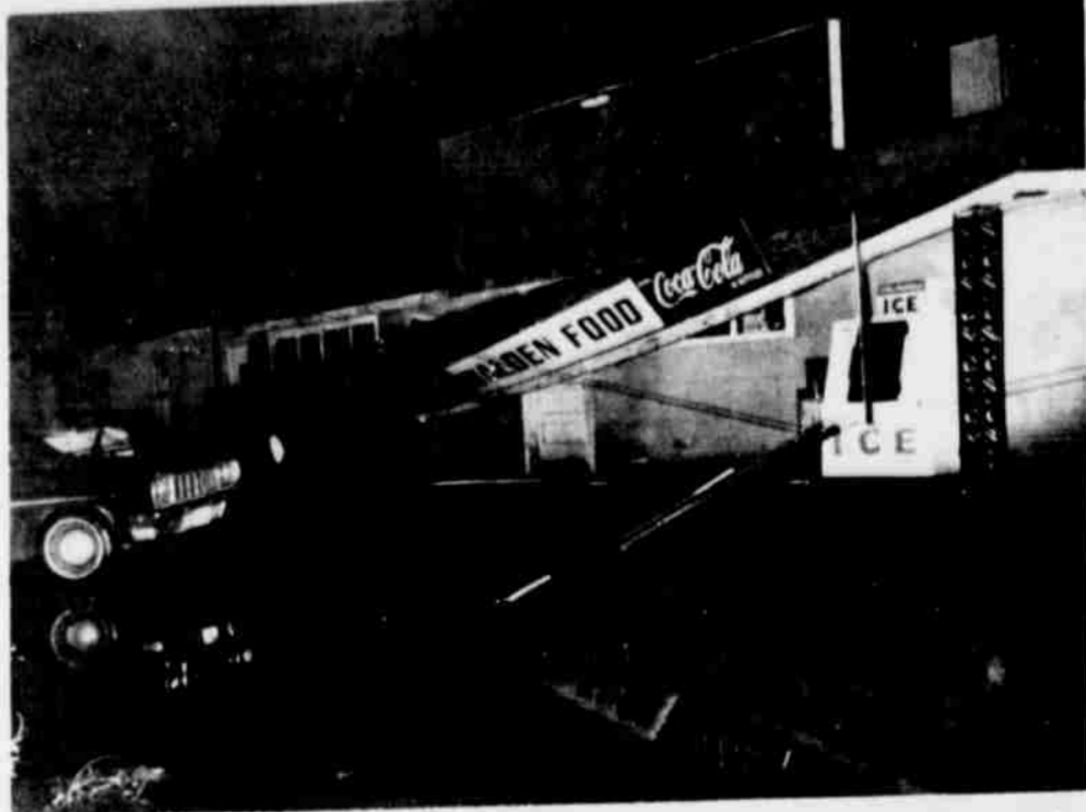
ELECTRICITY FROM power lines traveling up into the tornado that first struck at Walden's Grocery in Whitharral gave the effect of "a great ball of fire."
