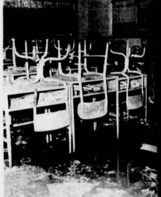
A MUD-CAKED, water-soaked and littered cafeteria on the south side of the Whitharral Elementary School shows some of the damage. The tornado day night was "dry" but the mud and water from the caved-in roof and rain following the twister.
