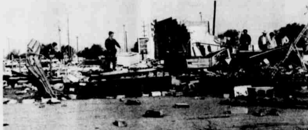
AG ADVISOR Omar Trip and some of his students look at what is left of the new concrete block agriculture building at Whitharral.
