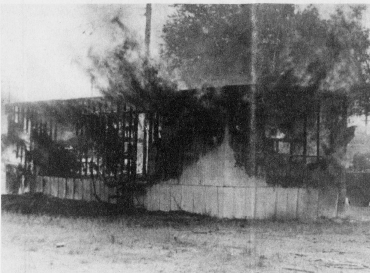
DEVASTATING FIRE---The trailer home of the Raymond Mendoza family on West Dallas Street was completely destroyed by fire last Tuesday afternoon. Jimmy Mills, Fire Marshal, stated that the fire apparently was ignited by a clothes dryer filter clogged with lint. (Journal Photo)
