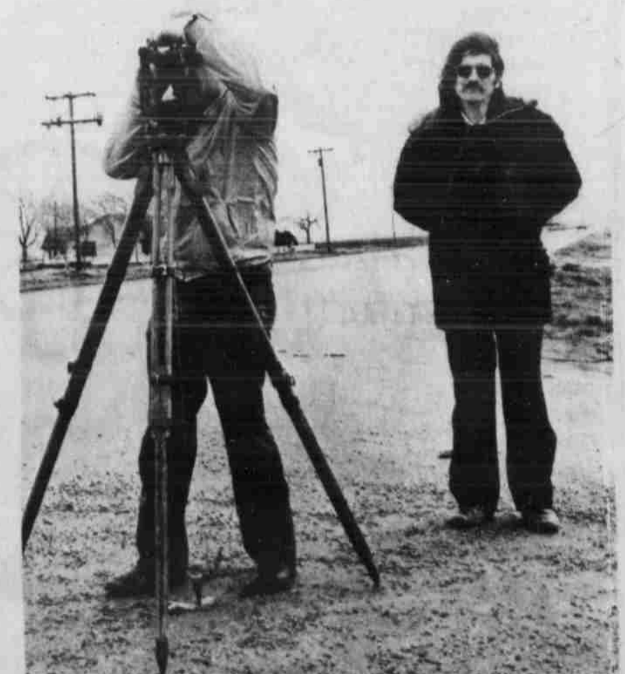
TOMMIE E. ANDERSON, registered public surveyor with Hugo Reed and Associates Land Surveyors of Lubbock, checks a measurement of the northern perimeter westward along the new textile and spinning mill site east of Littlefield Monday morning. Tuesday, a topography survey was begun. Aiding Anderson with the survey is Bob Smith. (Staff Photo)
