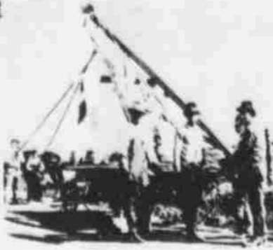
30 years ago the year Southern Public Service Company was born, raising transmission poles was literally a matter of horse and man power as pictured above. In the company's golden anniversary year, it's not a question of lift, set and tamp, as seen at right, nearly all of it done mechanically.
