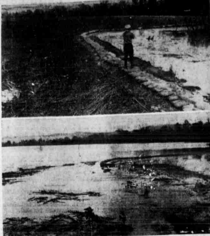
'BIG MUDDY' RUNS AMOK . . . Abnormal spring rains are causing floods in many parts of the country, inundating large tracts of land. Top panel shows the sandbagged levee of the Missouri river near Aldridge, Ill., before the rains came. Below, 36 hours later, the levee proves no barrier, the water breaking through to flood 2,000 acres of farm land.
