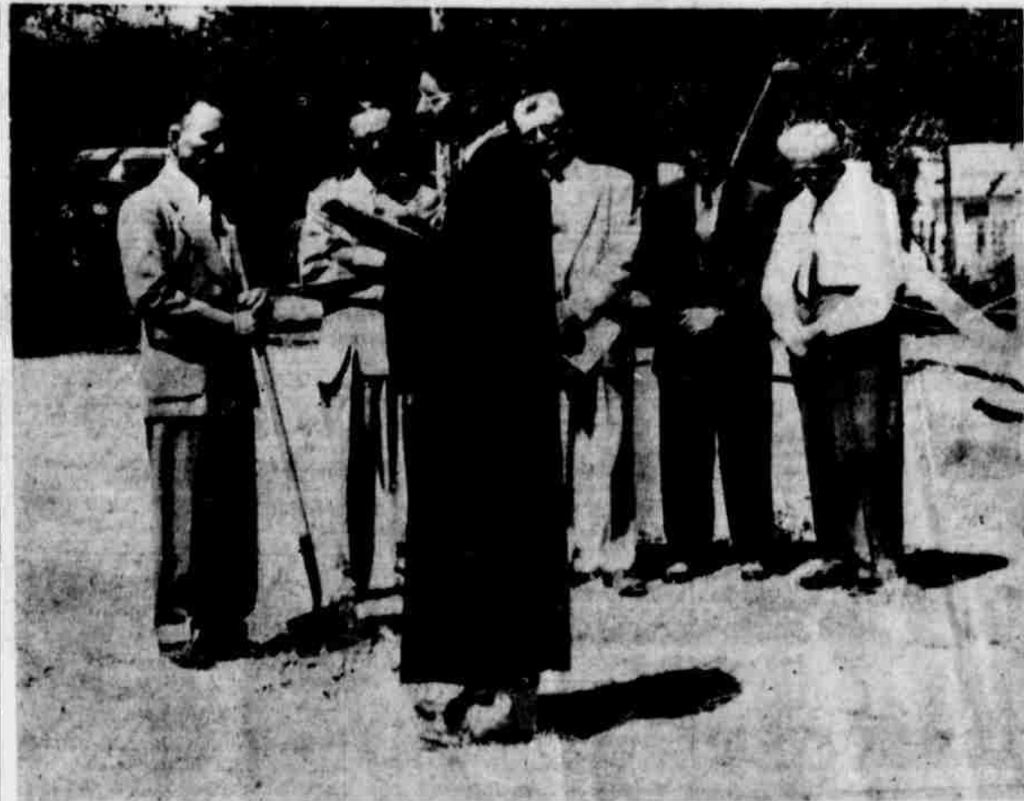
EMMANUEL LUTHERAN GROUND BREAKING for a new educational wing to be built behind the present Church structure. The groundbreaking was held Sunday morning as part of the regular service. Here, Pastor R. L. Young and members of the building committee take part in the special service. (Staff Photo)
