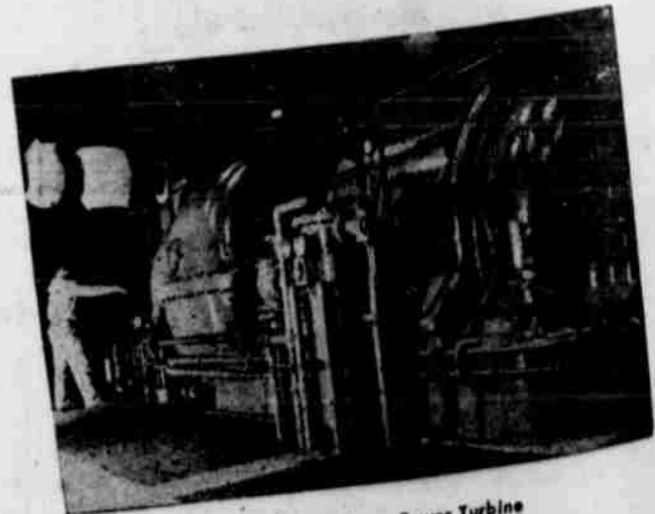
Giant 10,000 Horse Power Turbine
