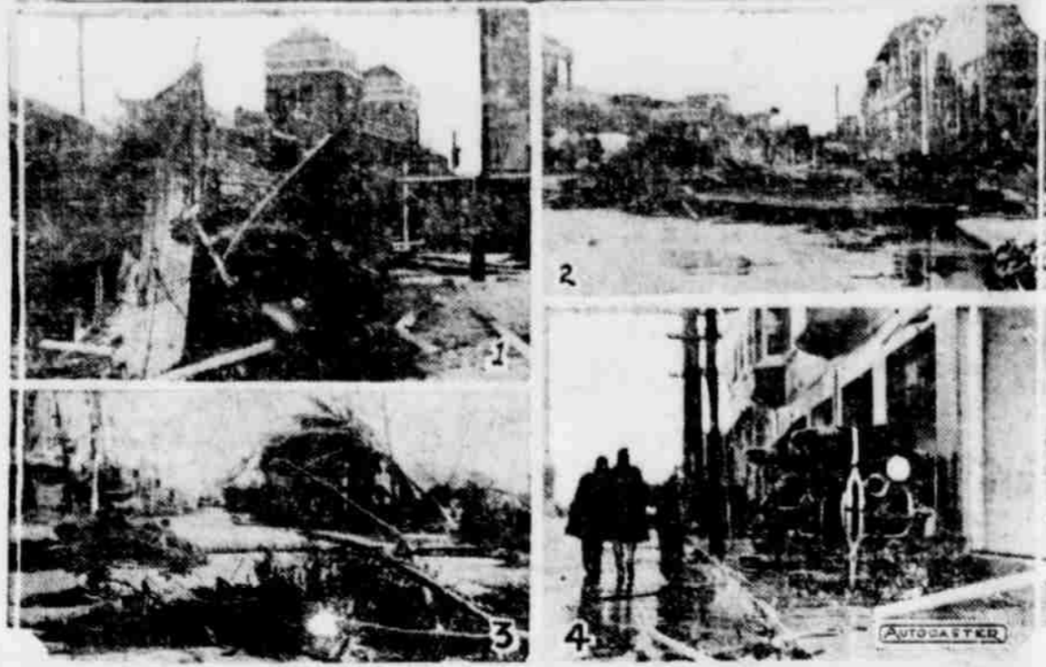
Two hours after the tornado had abated on the East coast of Florida these photos were northward bound by airplane, the first from the storm and wave torn districts. No. 1, Miami Beach front. No. 2, Fifth Street and Washington Ave. No. 3, Typical of great destruction which swept from east to north-west across the peninsula—tropical trees of ages crashing to earth. No. 4, The force of the storm shown in that 1½-ton motor car's position against the building. Loss of life not yet known.
