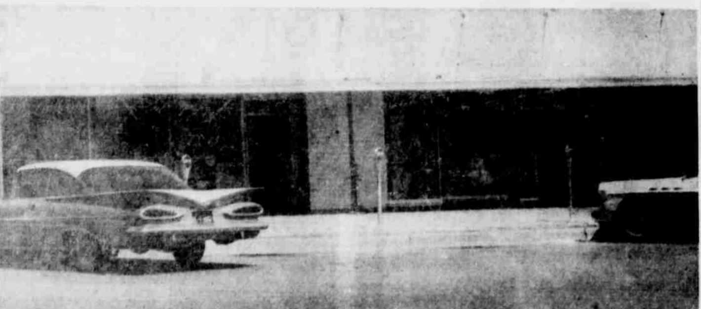
THE NEW FRONT . . . of the recently expanded Anthony store follows the style of the original front of tile and Kawneer aluminum with spacious glass installation for greater view into the store and window displays.
