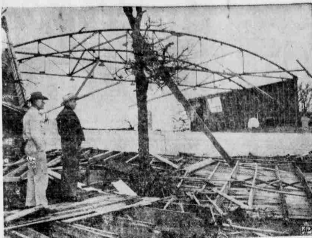
WIND-RUINED GYMNASIUM —A blast of wind ripped through the gymnasium at Smithfield Elementary School northeast of Fort Worth and left the structure without a roof and with east and west ends torn off. No one was injured as to "mad" winds struck the North Texas area. (AP Photo)
