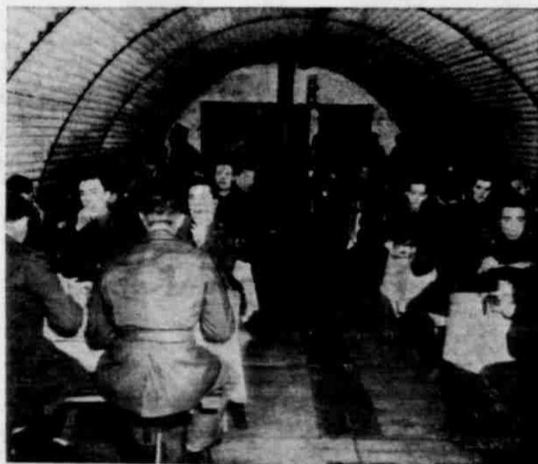
This photo, taken at one of Uncle Sam's strategic posts somewhere in Iceland, shows U. S. soldiers inside their mess hall, which is made of corrugated steel. "Our boys" are evidently enjoying their repast to the utmost.
