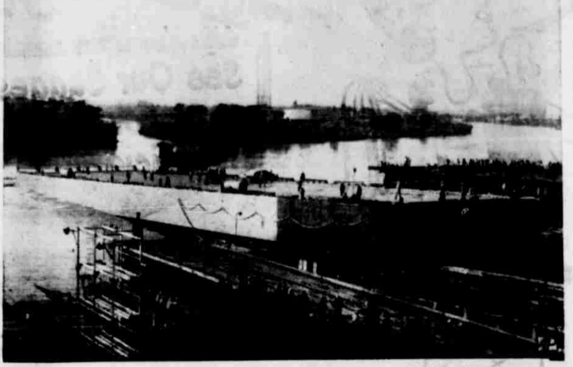
WORLD'S LARGEST — History's biggest steel dock barge was launched in Orange after it was built by the U.S. Steel Corporation at its plant there. The water vessel is 376 feet long and weighs 4 1/2 million pounds. It will be towed to Venezuela where it will be used in hauling ore on the Oranco River. —AP Photo
