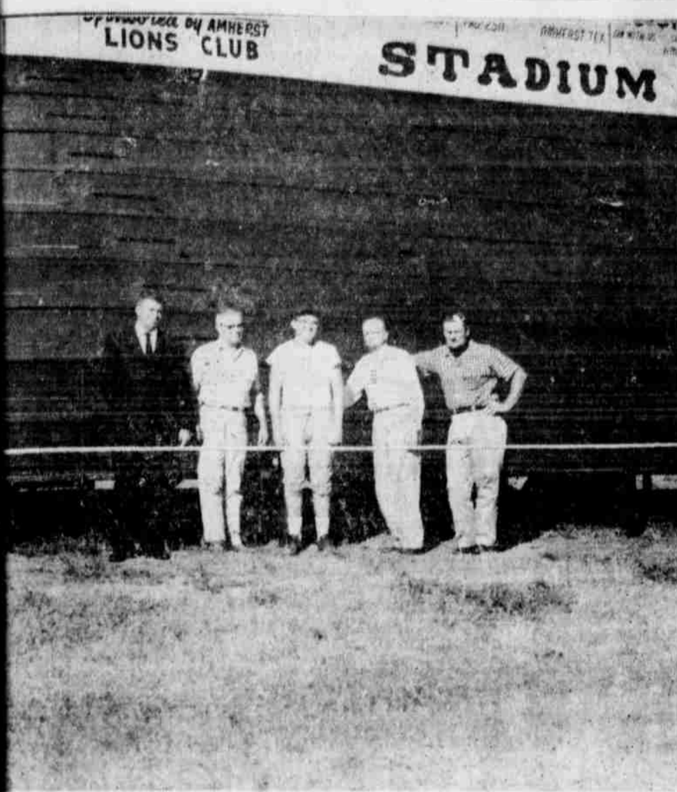
TAL, PAST AND PRESENT, in the building of Bulldog Stadium at Amherst are, C. L. Berry, principal of Amherst High School; Paul Bennett, president of the Amherst Bulldogs; Neal Chastain, head football coach of the Bulldogs; Elmer Watson, superintendent of Amherst school; and Arthur Hedges, head of the Lions Club building committee. (STAFF PHOTO)
