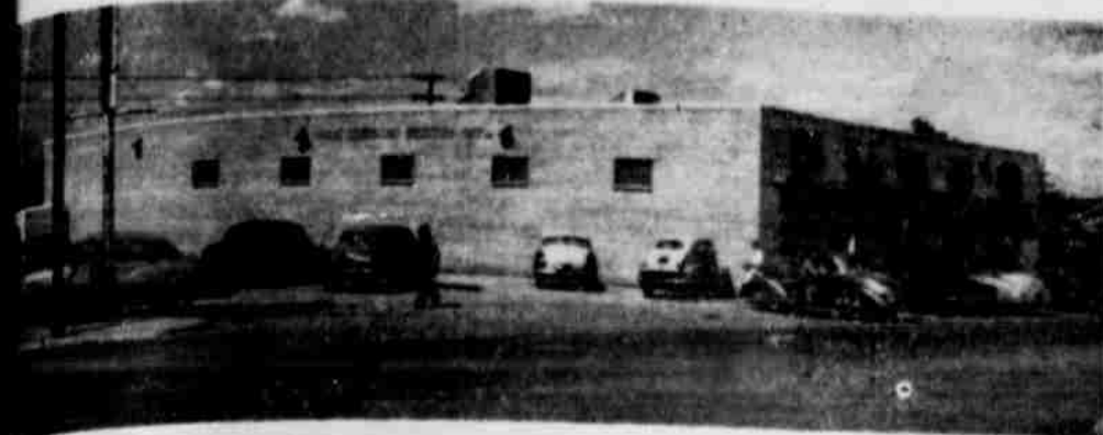
Here is a partial view of the Furr Super Market in Littlefield, with a section of the large parking lot for customers shown in the foreground. — Photo by NAIL
