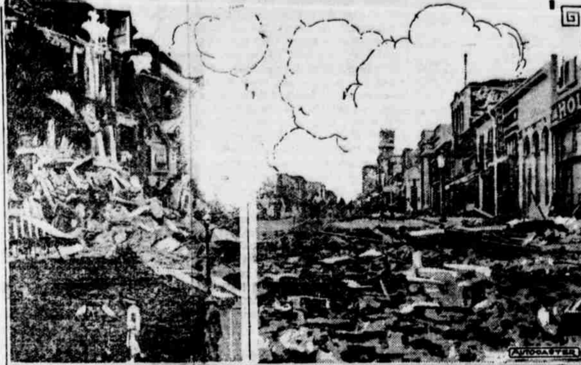
Here are two remarkable pictures, sent by telegraph, of the ruin in Santa Barbara, Calif., caused by the earthquake. At the left, the photo shows the ruins of the famous Arlington Hotel, almost completely wrecked. At the right—a view of State Street—principal business thoroughfare—as it looked one hour after the quake.
