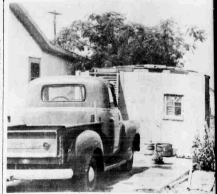
CARPOT TAKEN--The roof of a carport belonging to Oscar L. Sanders was lifted and scattered over a large area during the high winds Littlefield Sunday afternoon. The TV antenna on Sanders' house and the next door neighbor's were also claimed by the winds.
