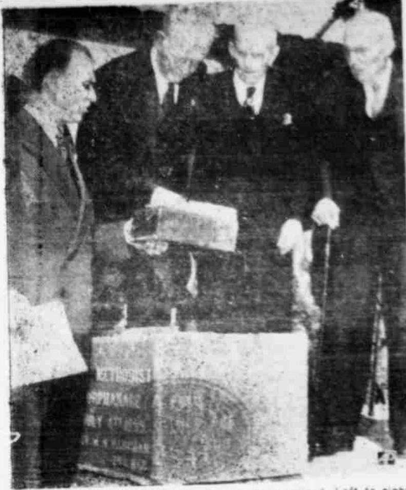
CORNERSTONE REMOVED — The cornerstone of the administration building at the Methodist home in Waco, Tex., has been removed and the 51-year-old
