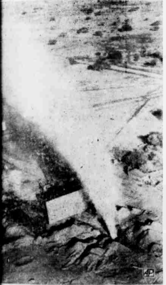
BLOWOUT —This salt water disposal well blew out one mile south of Bloomington, Tex., in Victoria County as it was being reworked and perforated in water sand at 4,000 feet. The Magnolia Petroleum Company attempted to stop the blowing gas and sand by perforating a twin well and pumping the sand full of mud. (AP Photo)
