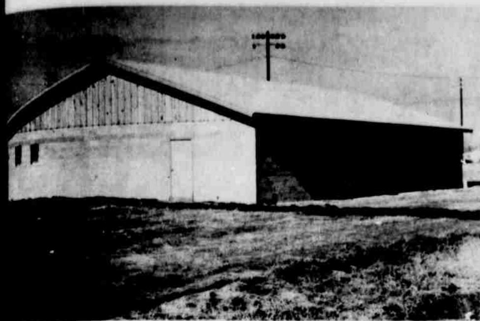
READY TO OPEN -- Pictured above is the new Jaycee building on the Fair Grounds which will officially open New Year's Eve with a dance. (See story on Page One).
