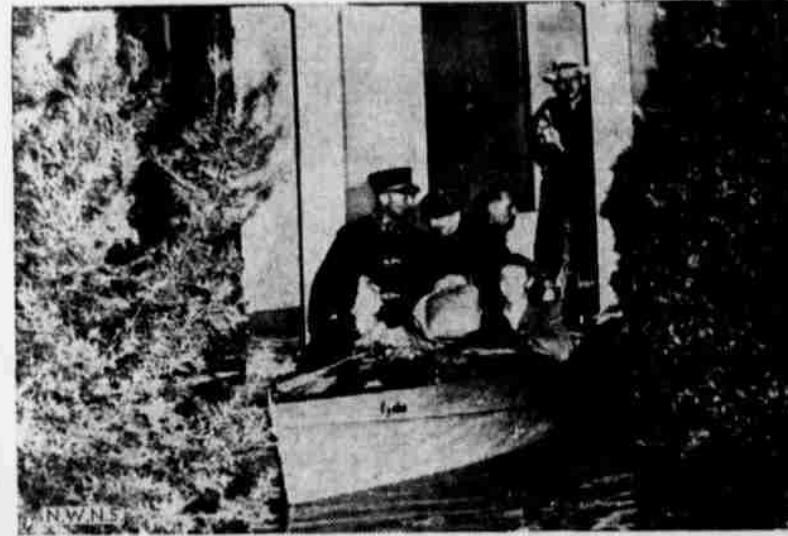
A broken dike released this flood on the streets of Hutchinson, Kas., when Cow creek, raging after heavy rains broke through retaining walls. This photo shows occupants of a house in the residential district as they were evacuated by boat after having been marooned for several hours
