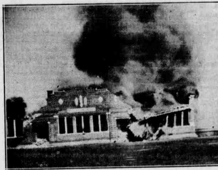
Above are two photographs of the fire which destroyed the Pep School Christmas morning. A teacherage was constructed recently to be used as a school for the remainder of the current term. Plans are going forward for a new and modern school building. The photographs, which are here reproduced, were taken by J. E. Stengel, a member of the Pep school board, who obtained his camera immediately after he observed that it would be impossible to extinguish the blaze.
