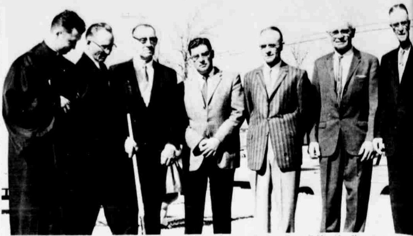
GROUND BREAKING CEREMONIES at the Emmanuel Lutheran Church in Littlefield included the pastor of the church and building committee, who each took the spade. Left to right they
