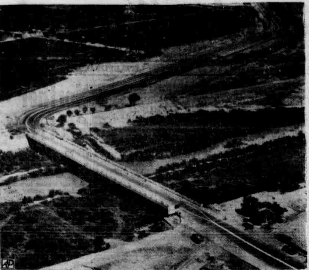
NEW INTERNATIONAL GATEWAY —Air view from Mexican side of Rio Grande shows bridge and roadway of first major U.S.-Mexico port of entry to be opened in over 70 years. Immigration center is in triangular area at upper right, and U. S. soil just beyond. Over 20 years of fruitless negotiations preceded successful break of log jam to provide second bridge at El Paso at the largest U. S. entry port, with 25 million entrants per year. (AP PHOTO)
