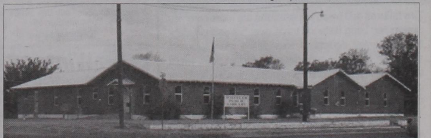
NEW WINDOWS: The City of Wheeler recently had new windows installed in the Wheeler Public Library at the corner of Hwy. 152 and Canadian Street. The structure was built for use as a hospital by Dr. H. E. Nicholson in 1942. After the deaths of both Dr. H. E. Nicholson and Dr. Harold Nicholson, the building was given to the City of Wheeler for use as Library. After undergoing some remodeling after being donated, the building presently houses the library and Wheeler Girl Scouts.
