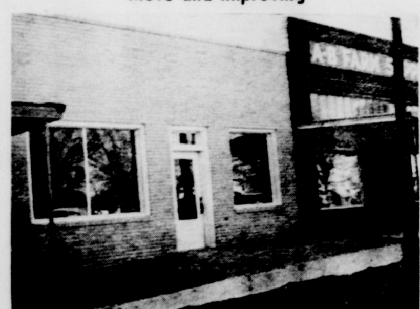
ATTORNEY OFFICE: D. O. Beene, attorney at law in Wheeler, recently completed construction and has moved into this new building. The building is located next to the A and B Farm Supply.
