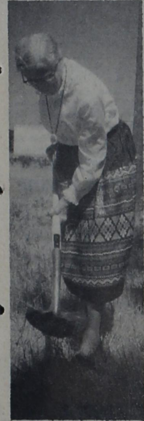
FIRST SHOVEL OF DIRT: Esther Sorensen, a Wheeler County Pioneer had the honor of turning the first shovel of dirt at the ground breaking ceremonies for the new First National Bank in Wheeler. The ceremonies were held Tuesday June 14. Chuck Hogan, director, observes.
