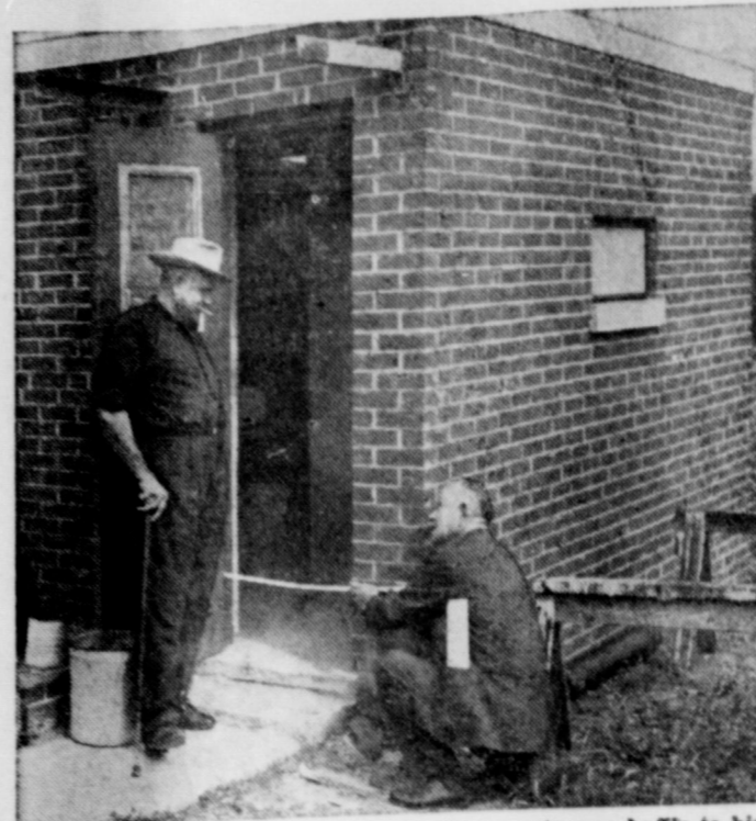
ENGINEERING ADVICE on how to add an entrance baffle to his new fallout shelter is obtained by Carl L. Underhill (left), of North Raleigh, N. C., from Archie W. Green, Jr., engineer for the North Carolina Civil Defense Agency. Underhill discovered that a baffle was needed to block dangerous levels of radiation which, after nuclear attack, could penetrate a normal door of this $1,000 shelter. Green was hired early in 1961 under a Federal program to pay half the costs of new civil defense employees. (OCDM Photo)
