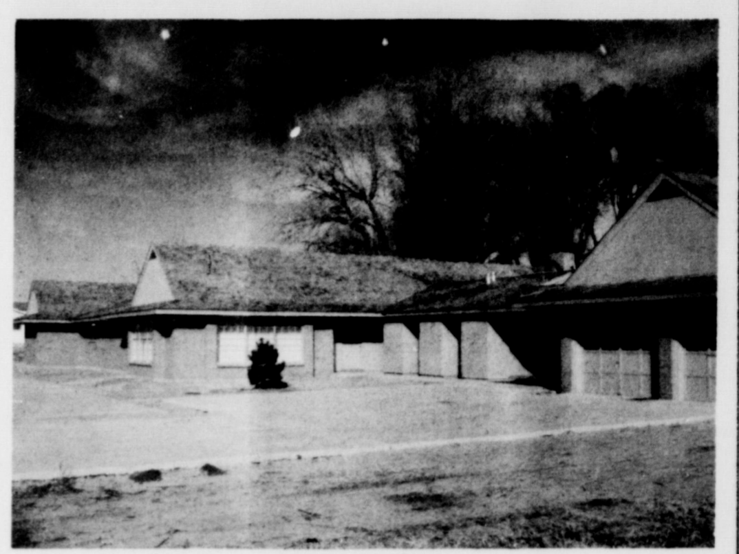
THE BARTON HOME: Mr. and Mrs. G.C. (Chief) Barton moved into this new home shortly before Christmas. Contained in the home is 3120 sq. ft. This area is broken up into three bedrooms, three baths, utility, kitchen, dining room, family room, and living room; a hobby room is located behind the two car garage. The house is 140 ft. 10 in. long and is located on Stanley street. Styled Country French, the exterior is done in Tree Bark Gary brick and wood. Featuring a dooburn-ing fireplace, the family room and dining room has an open-beam ceiling with Chicago Brick being used in the fireplace and kitchen. The paneling and cabinets are of ash. The furnishings are of antique and colonial. A dining terrace is enclosed on three sides by the living room, dining room and entrance, the living and dining rooms open onto the terrace. The home is centrally heated with gas.
