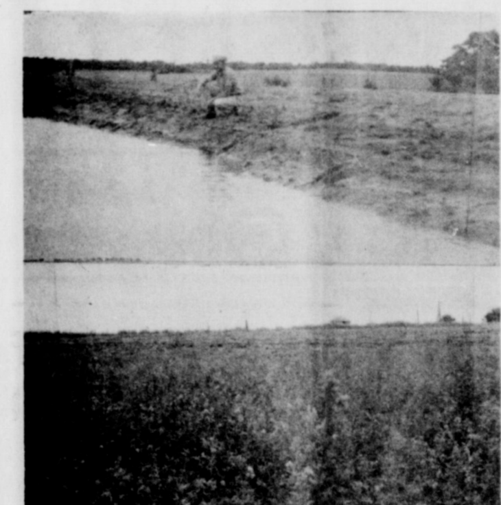
H.D. Pond of the S.C.S. is shown on a diversion terrace constructed this year by J.H. Williams. The diversion on which Pond is sitting is protecting a field of alfalfa from excessive runoff from a hillside above.
