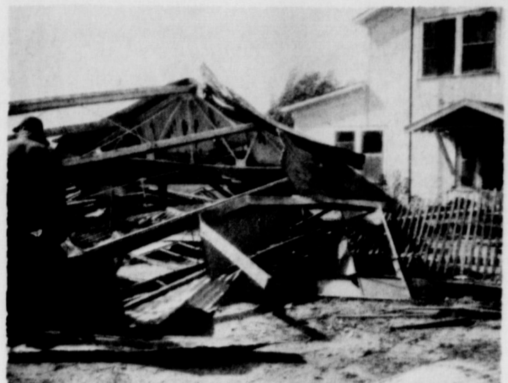
WIND DAMAGE: Two Gageby community residences received wind damage late Wednesday evening. A steel shed, recently moved to the Wayne Meek farm, was moved across the yard and left destroyed just a few feet from the house where the family was at the time of the storm. A chicken house and the windmill wheel were also destroyed at the Meek farm. Three buildings received damage at the Farmer Hefley farm two miles south of the Meek farm. Three windows were broken in the house, one side of the garage was torn from the foundation and a chicken house was flattened. The storm struck between 11:00 and 12:00 and caught everyone asleep. Mr. Meek was looking out at the clouds when the storm struck. The building destroyed at the Meeks was piled on top of the cellar.
