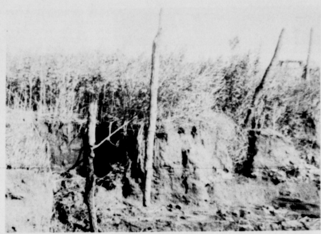
FAMILIAR SIGHT? This producer solved his problem by installing a concrete chute. This type of structure stopped a gully from cutting a valuable field in half. If you have an erosion problem contact your Wheeler County Soil Conservation office.
