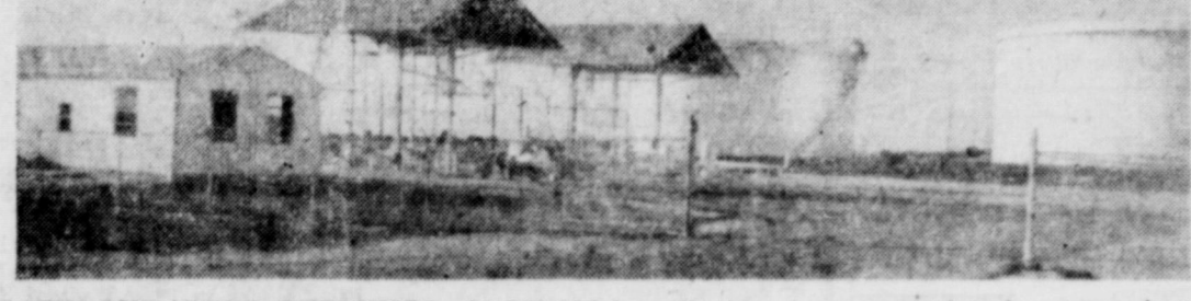
EASTLAND GULF TERMINAL. $1,500,000 installation just completed near here. Charles Turner, who has opened several terminals, is in charge as superintendent.
