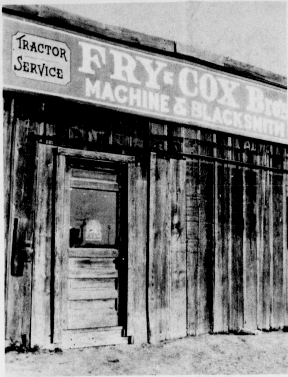
YOU'VE COME A LONG WAY - - - Pictured is the original building which housed Fry and Cox Bros. Machine and Blacksmith Shop at the corner of Main Street and American Blvd. where St. Clair's parking lot is presently located. This week, Fry and Cox Implement will be celebrating 50 years of service and continuous business in Muleshoe. They are located at the corner of West First and West Avenue D, Jack Cox, and his son, Edwin, present operators of the business, will hold a special celebration sale, plus present a number of prizes.
