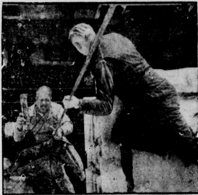
PREVENTING A HEADACHE— Steeplejack Ralph Clark, his dangerous task completed, is hoisted back to the roof of a San Francisco hotel. Clark was suspended by rope 13 stories above the street to remove a loose chunk of concrete before it could fall and cause damage. Looking down from the hotel's roof is Clark's helper, Ernest Pigge.
