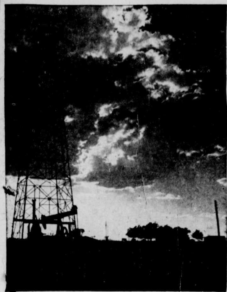
A DISAPPEARING SCENE —Derricks such as these are in the twilight of a fabulous career. In the past derricks were left at well locations for use if it was necessary to work over the well in the future. Now a portable workover rig is in general use. This derrick, near Big Spring, Texas, will probably be torn down as will many others like it as the industry moves ahead into another year of progress.
