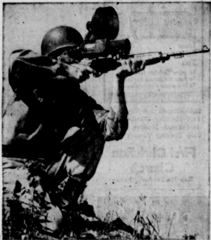
NIGHT SIGHTING. An Army sharpshooter sights through the new infrared "sniperscope." The new sight, an improvement over its World War II predecessor, can spot an enemy at night at a much greater distance. The power supply is carried in a lightweight cartridge belt container instead of in a cumbersome back pack. Developed by Raytheon Company for Army's Engineer Research and Development Laboratories, the "sniperscope" is scheduled for large scale production in the near future.
