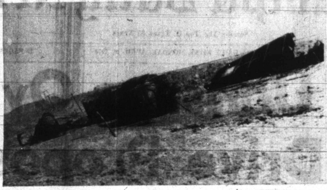
THESE ARE a part of six railroad cars the twister left near J. 40 three miles west of McLean. One car appeared to be ready to make a trip down a dirt road and enter the highway. Railroad tracks were not visible to the Pampa Daily News photographer. (Staff Photo)
