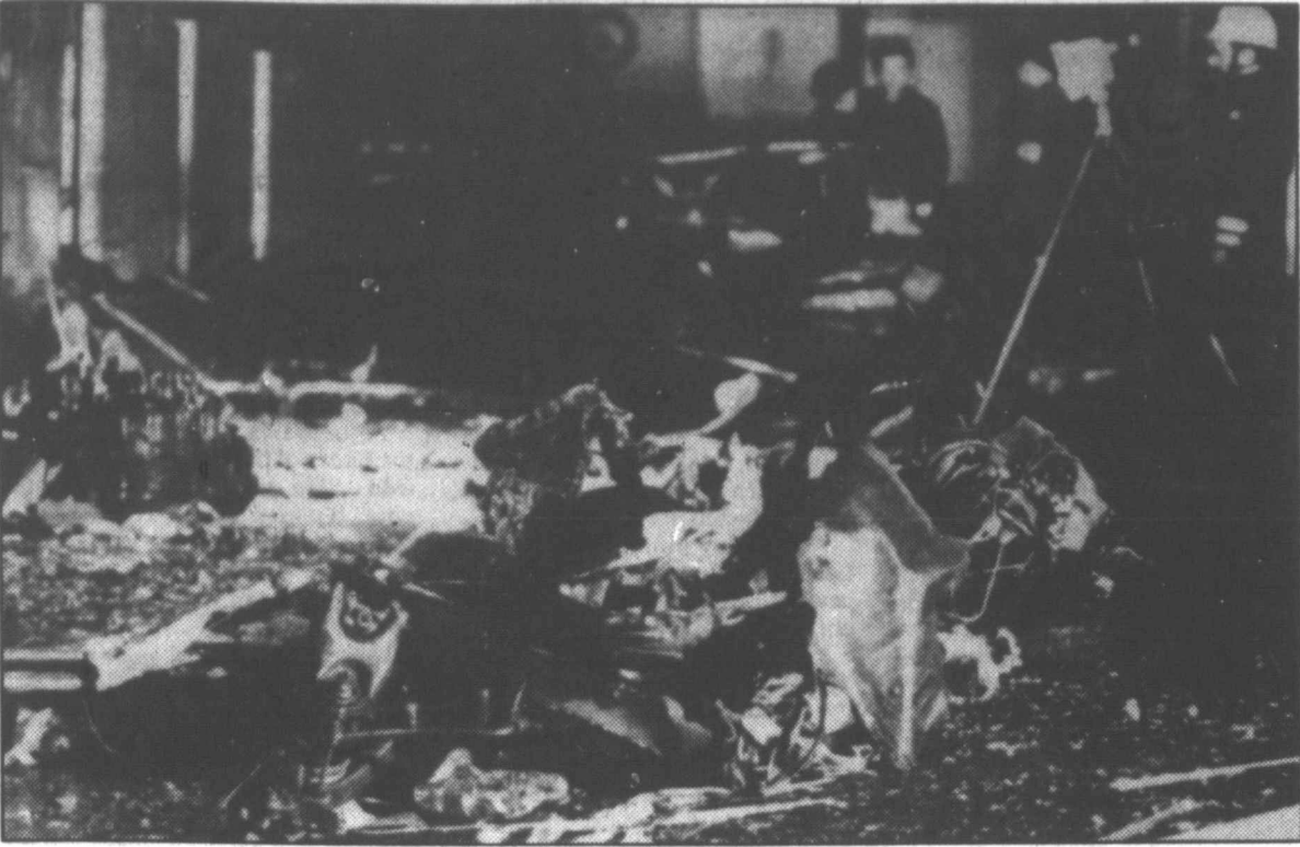
BOMB SCENE —A car parked in front of the Belgian Employers Federation building in Brussels exploded early Wednesday killing one fireman, injuring 13 other people and causing heavy damages to surrounding buildings. Remains of the car are in the foreground. The explosion is claimed by the left-wing terrorist group "Cellules Communistes Combattantes."
