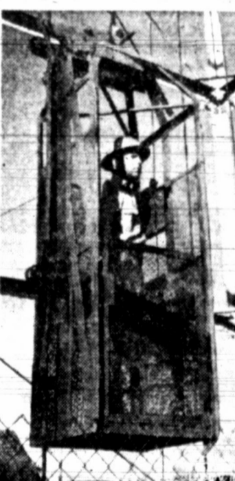
NO MORE HUFFING —Forest fire lookout has it made on a tree farm near Molalla, Ore. Elevator bypasses those long, long stairs as a means to get to top of the 140-foot tower.
