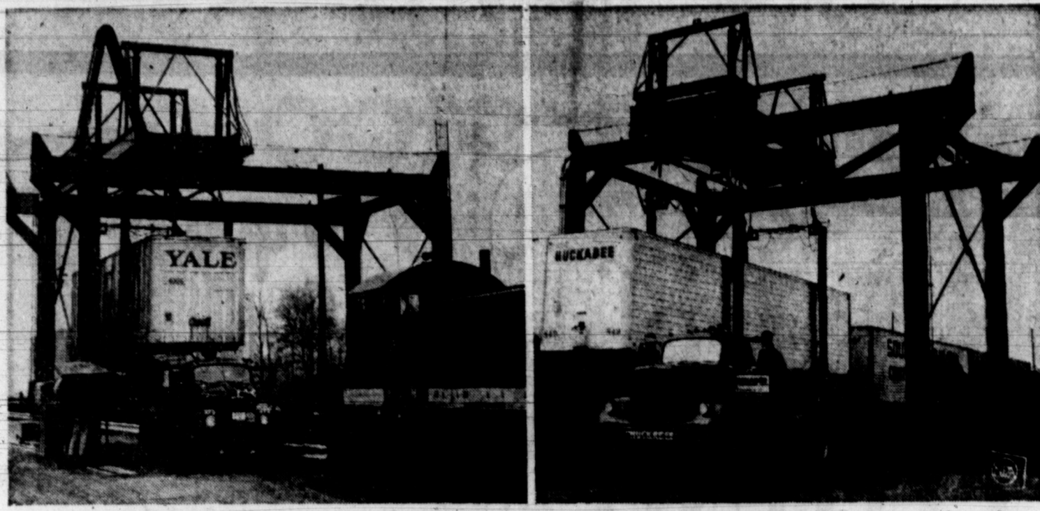
HOW IT'S DONE —Ever wonder how those truck trailers get on top of those piggyback freight cars? The circuses used to roll their wagons up a ramp on the end car and then over between-car bridges until they reached the
